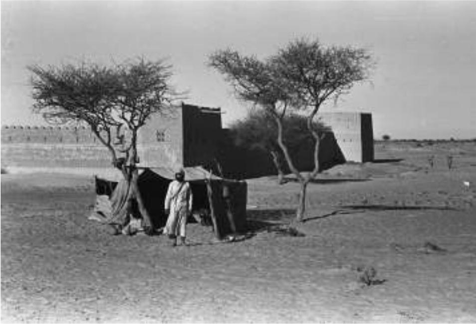
Fig. 3 – The north wall of Muwaiji Fort photographed by Thesiger in 1948-49. The north-east tower (left of centre) appears to have formed one of the living quarters of the fort prior to the occupancy of Shaikh Zāyid. The photograph also shows that no rooms had been added to the tower at this date, and thus that these were a later feature added by Shaikh Zāyid.
