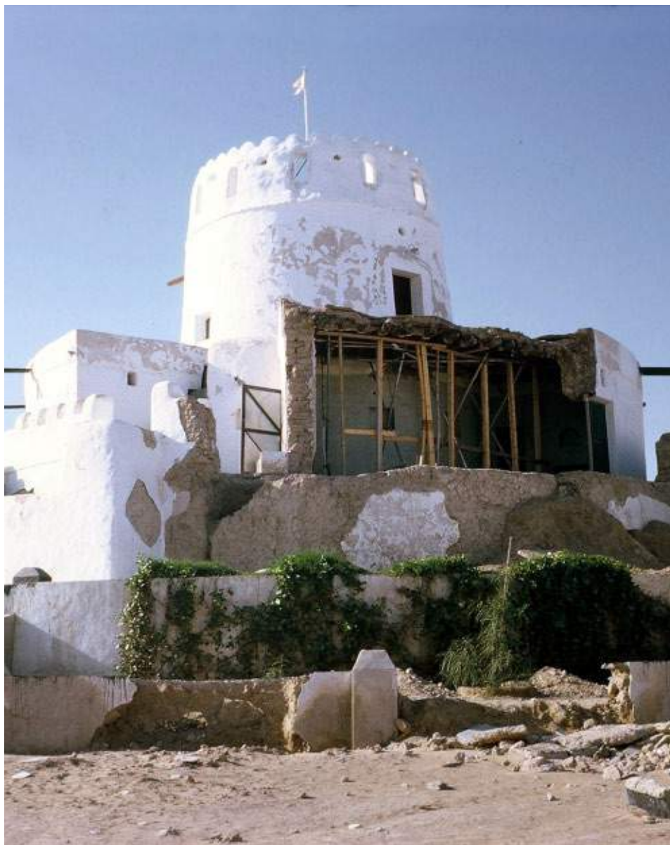
Fig 14 This startling view of the round watchtower with the officers' quarters and mess was taken just after a devastating rainstorm had caused the collapse of some of these additional mud rooms. Postern gates let in to the enclosure wall to provide access to the exterior of the fort can be seen at the right and left of the picture. Col. Edward Wilson © TCA Abu Dhabi.
