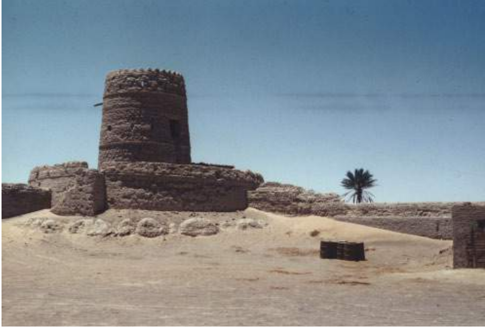
Fig 4 Peter Clayton's view of the watchtower taken in March 1956, showing the original entrance set high in the wall, as well as the steps leading to the top of the revetment around the tower. The photograph also shows drifts of sand against the inner face of the enclosure wall with a recessed wall walk. © Peter Clayton.
